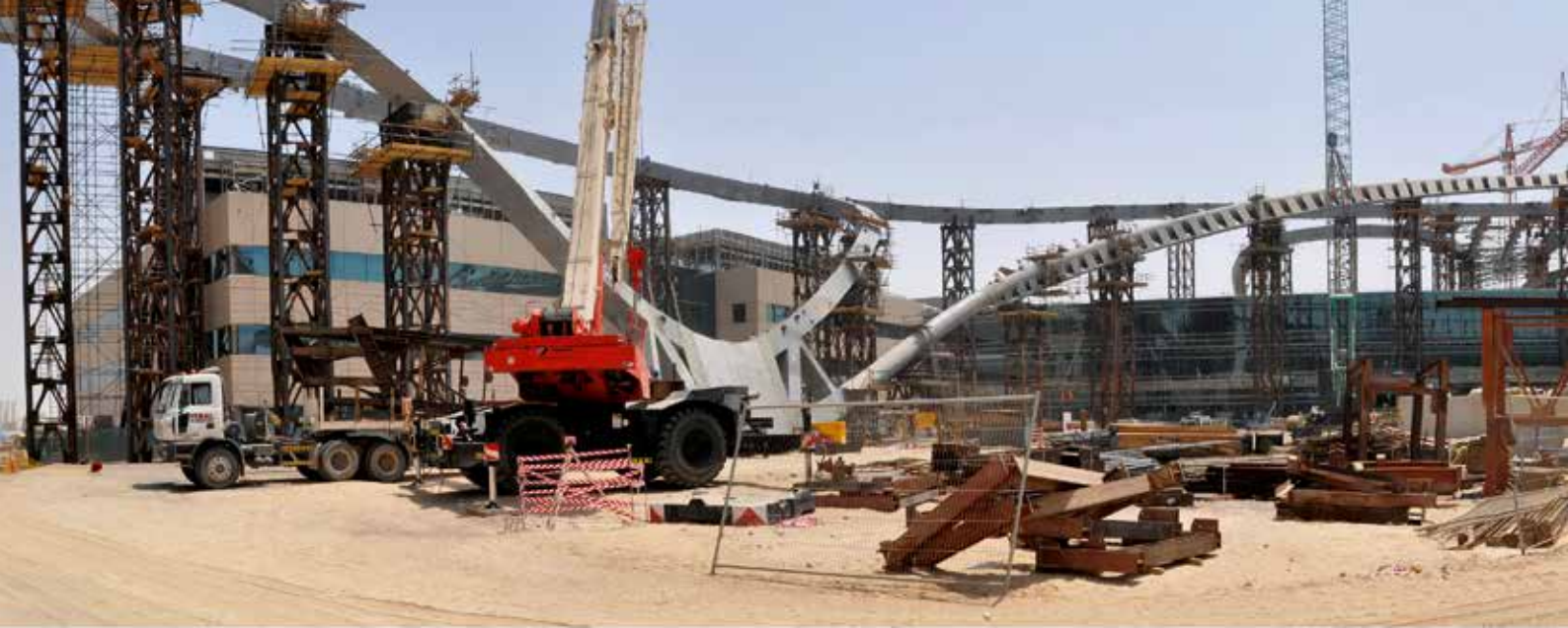
Erection of the secondary steel structure subsequent to primary ring structure
