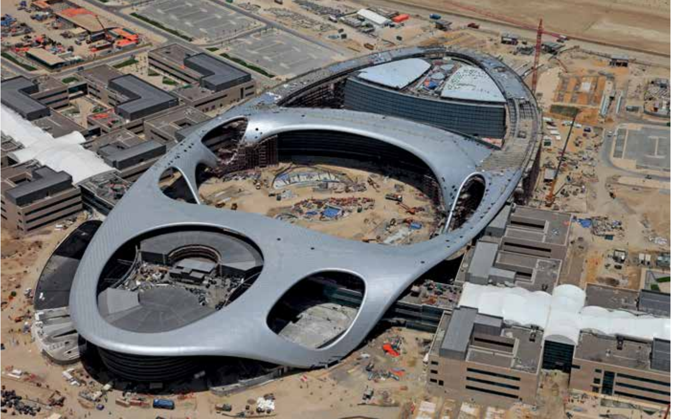
Central Feature Roof under construction
