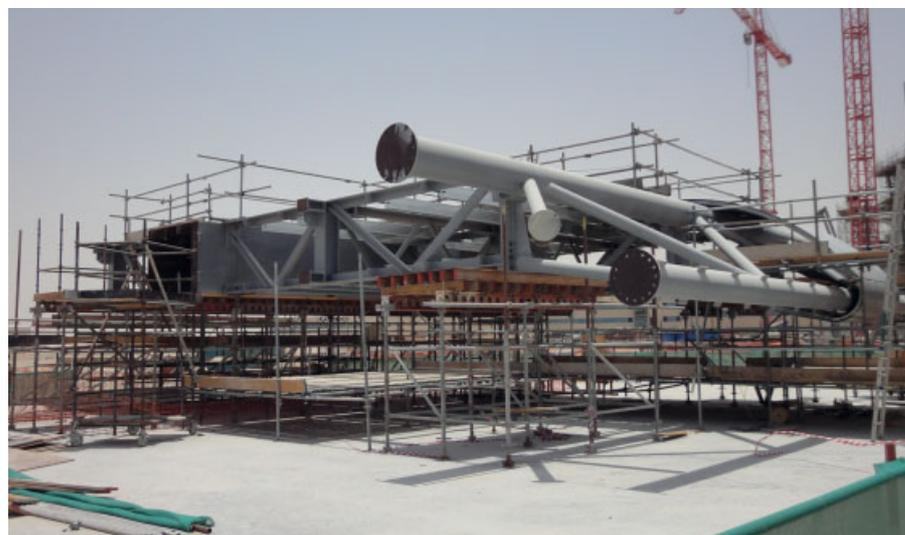
Fig. 15. Mock-up for steel structure and cladding
