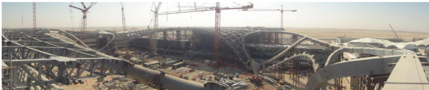
Fig. 13. Erection of the secondary structure subsequent to primary ring structure
