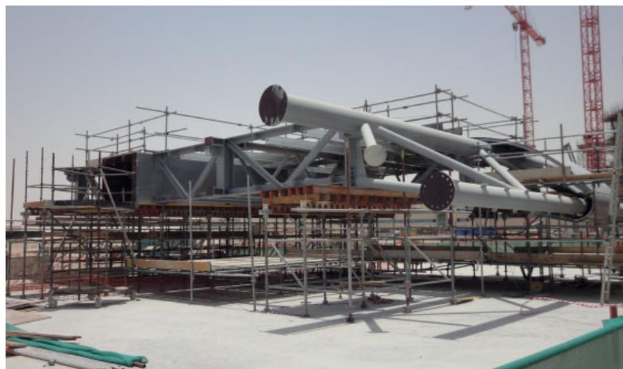
Fig. 15. Mock-up for steel structure and cladding
